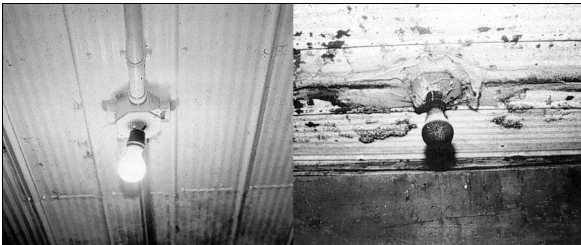
FIGURE 2. Low cost incandescent systems have high maintenance and operating costs. Note the dirty build-up on a long-life lamp.
