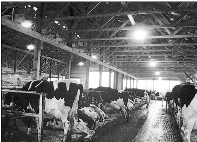
FIGURE 8. High pressure sodium fixtures (the light is yellow). (Source: Agviro, Inc.)
